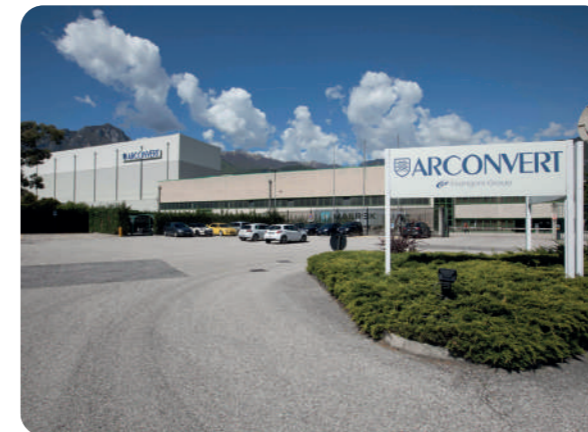
Automated self-supporting storage system (paper sector)
