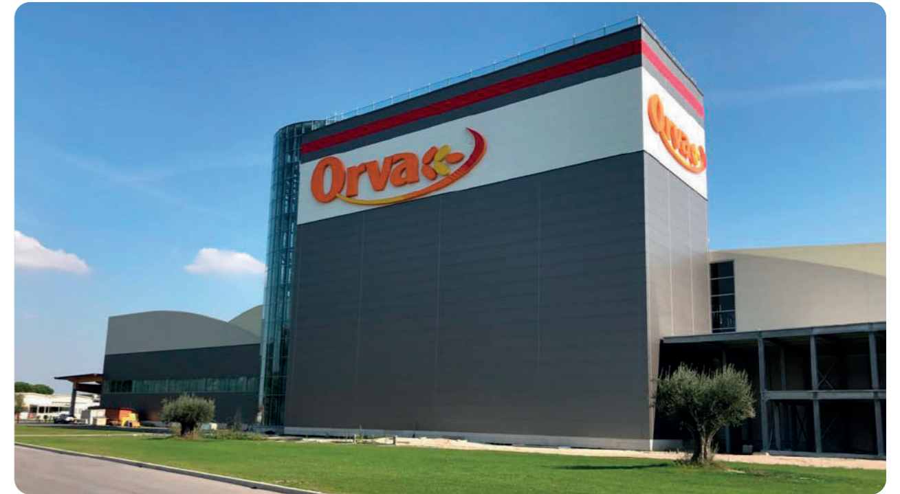
Automated self-supporting storage system (food and beverage sector)
