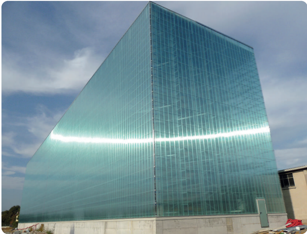
Automated self-supporting storage system with polycarbonate panels (mechanical sector)
